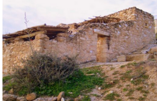
An Israelite home built into the limestone slopes of the Judean hill country near Bethlehem. Homes were often constructed around existing natural features like caves
